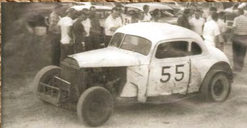
Bennett raced this Hudson Coupe from 1963 to 1965, breaking track records with its combination of a Hornett engine and light weight.
